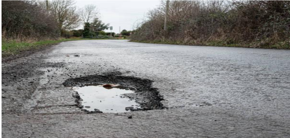
Figure 8 Precipitation-induced pothole [50]
