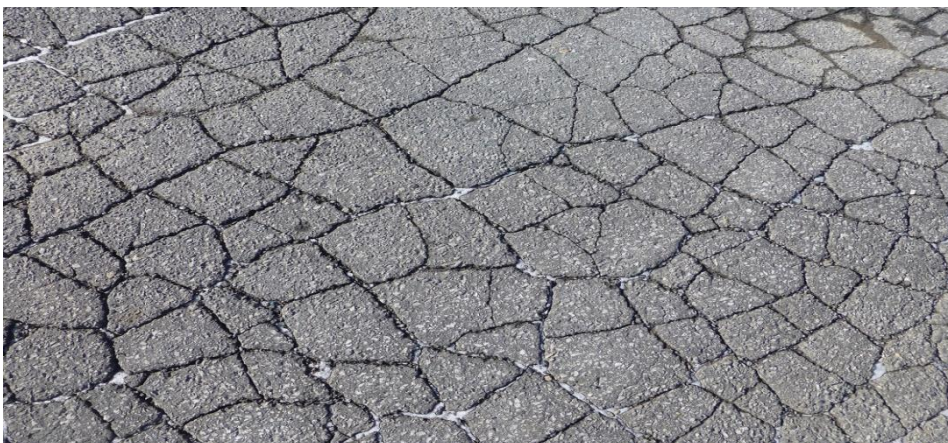
Figure 5 Thermal cracking [40]
