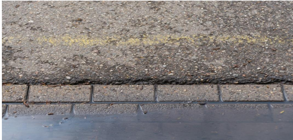
Figure 6 Pavement spalling [43]
