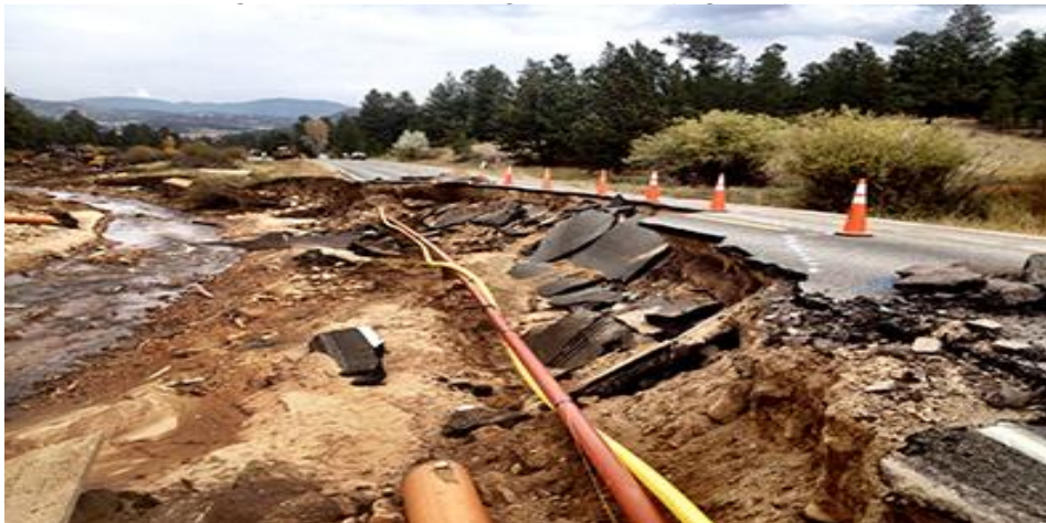
Figure 9 Precipitation-induced erosion [53]
