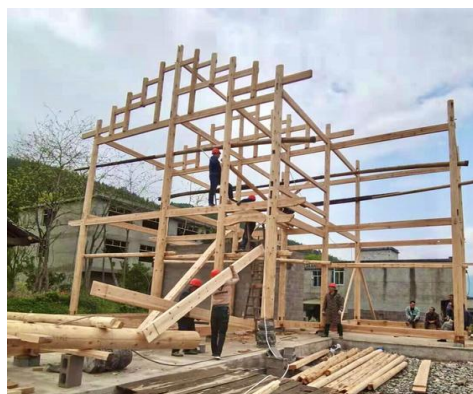
Figure 17: The Wooden Constructive Structure of the Dong Building
